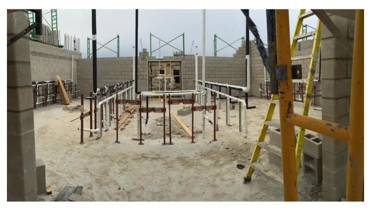
WALLS - Block walls are being erected at the Gymnasiums. Plumbing rough-in is being installed at the student restrooms.
