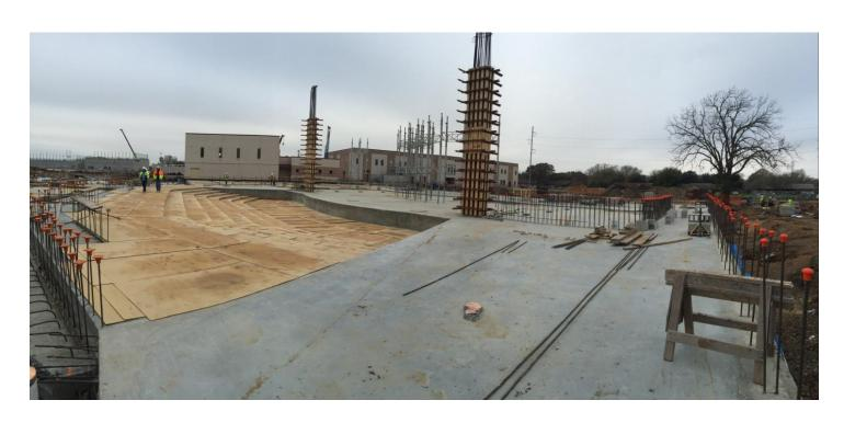
**FOUNDATION** – Foundation has been poured at the Auditorium Stage and Seating Area in front of the Stage. The plywood at the stepped seating area is used for concrete floor protection. The two columns at either side of the stage will support the concrete beam that spans the stage opening.
